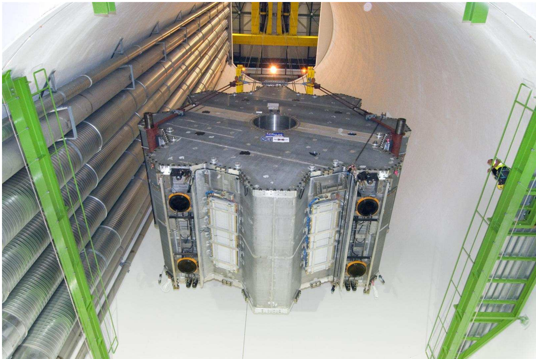
Figure 3.11: The ATLAS end-cap toroid being lowered into the cavern[30]
